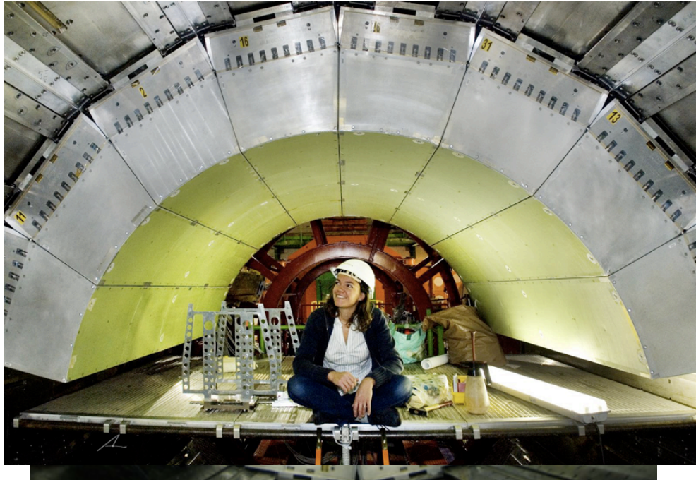
Central ECAL installation in CMS
