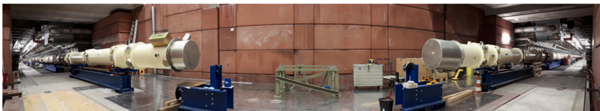
A schematic view of the ALPS-II layout with its 24 dipole magnets (top), and a recent view of the HERA tunnel, with 12 magnets installed on either side of the future central region of the experiment, seen through a fisheye lens.
