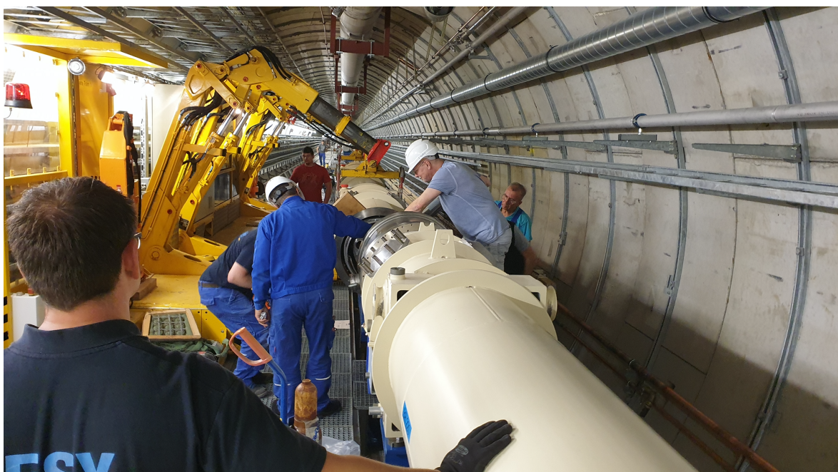
The ongoing installation of dipoles for ALPS II in the former HERA tunnel at DESY.
