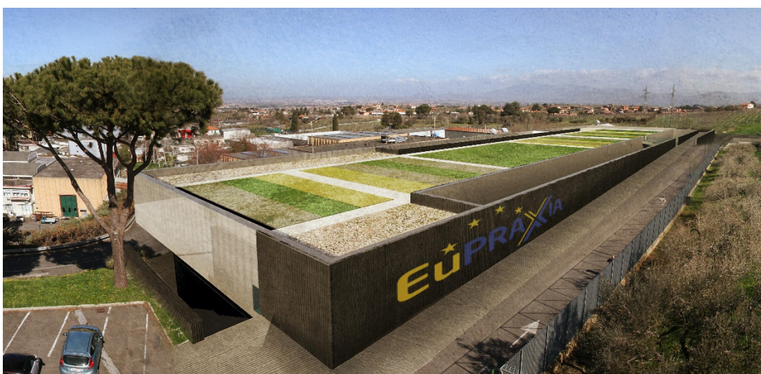
3D-rendering of the EuPRAXIA construction site at INFN-LNF. The design process of the building has recently started, it will have dimensions of 134m x 35m with a potential extension added at a later point (image credits: Simona Incremona, General Services and Technical Division).
