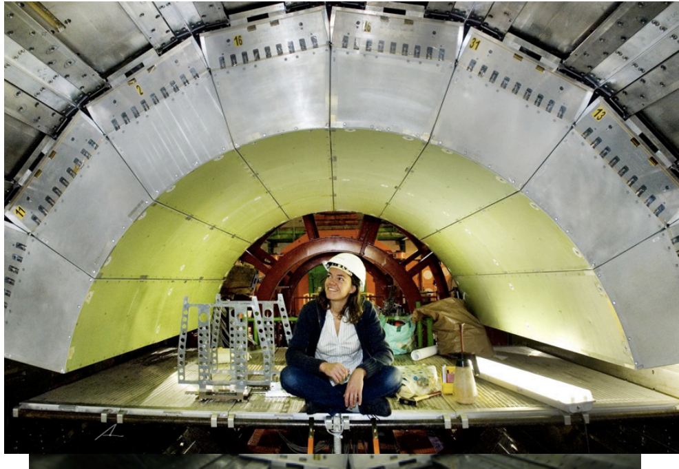
Central ECAL installation in CMS
